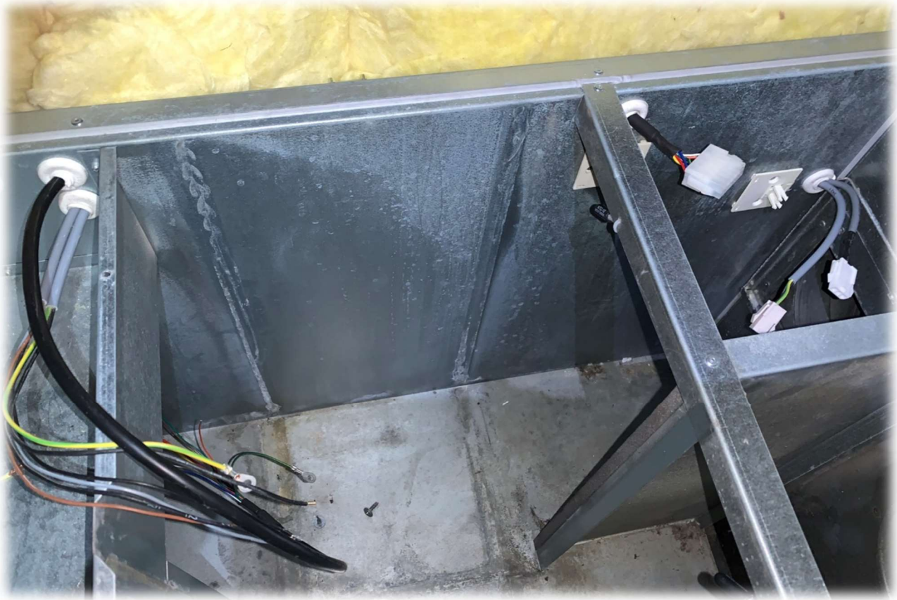
New cables installed.
