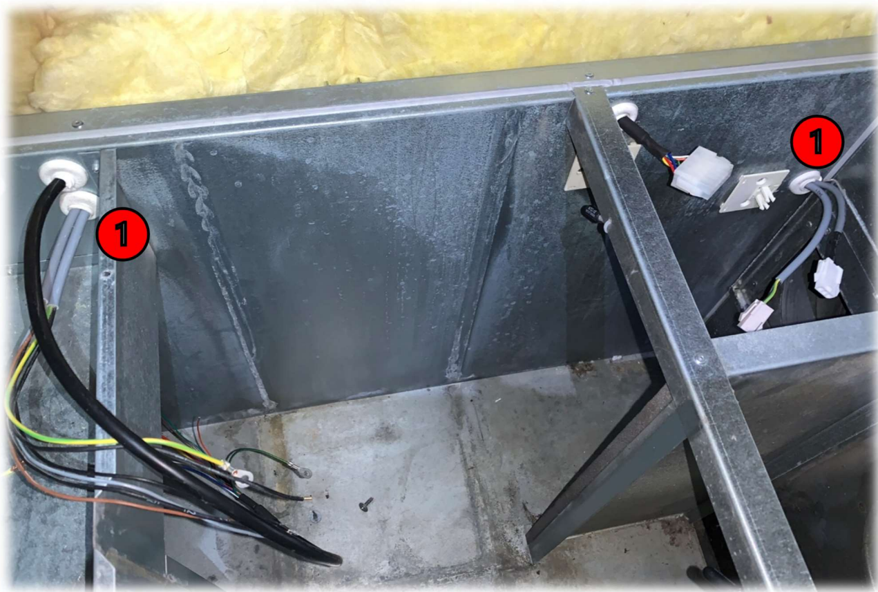
New extract air fan cables installed (1).
