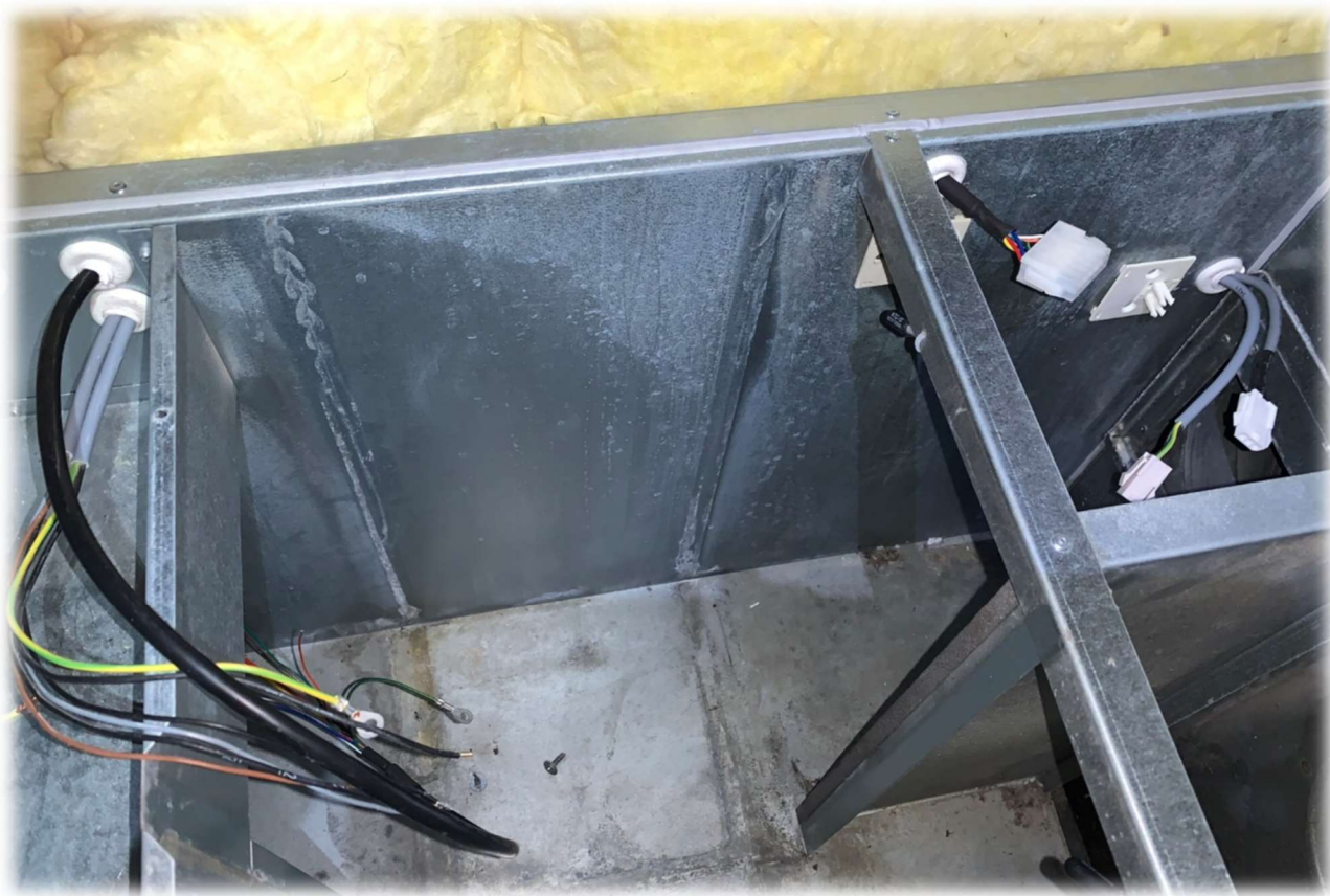
New cables installed.
