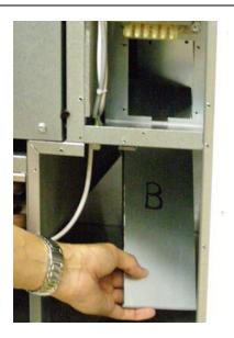
Keep damper B in the air lifted through the hatch and pull/press it firmly towards you while drilling screws through the rear wall of the switchboard screws into damper B (3 pcs).
