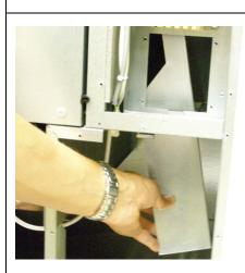
Insert damper "A" into the supply air duct.
