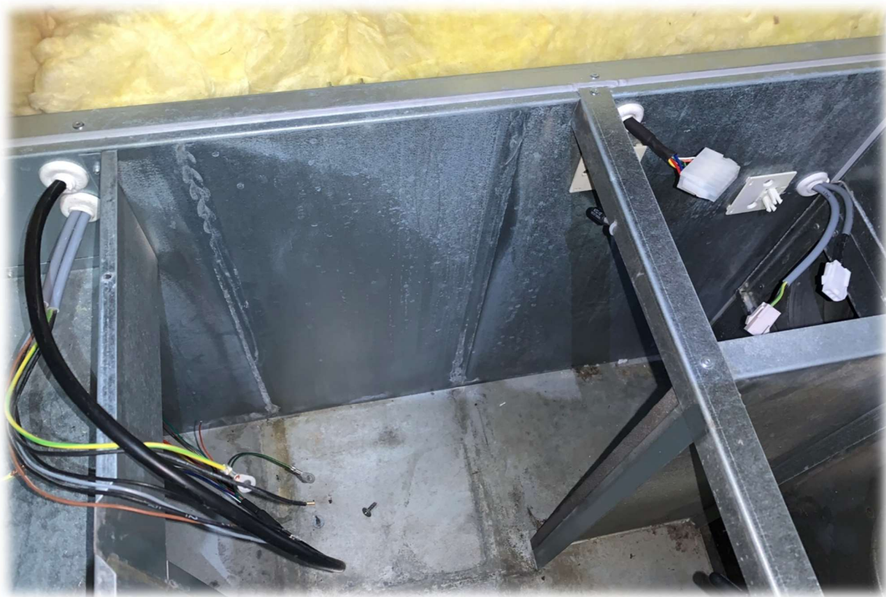
New cables installed.
