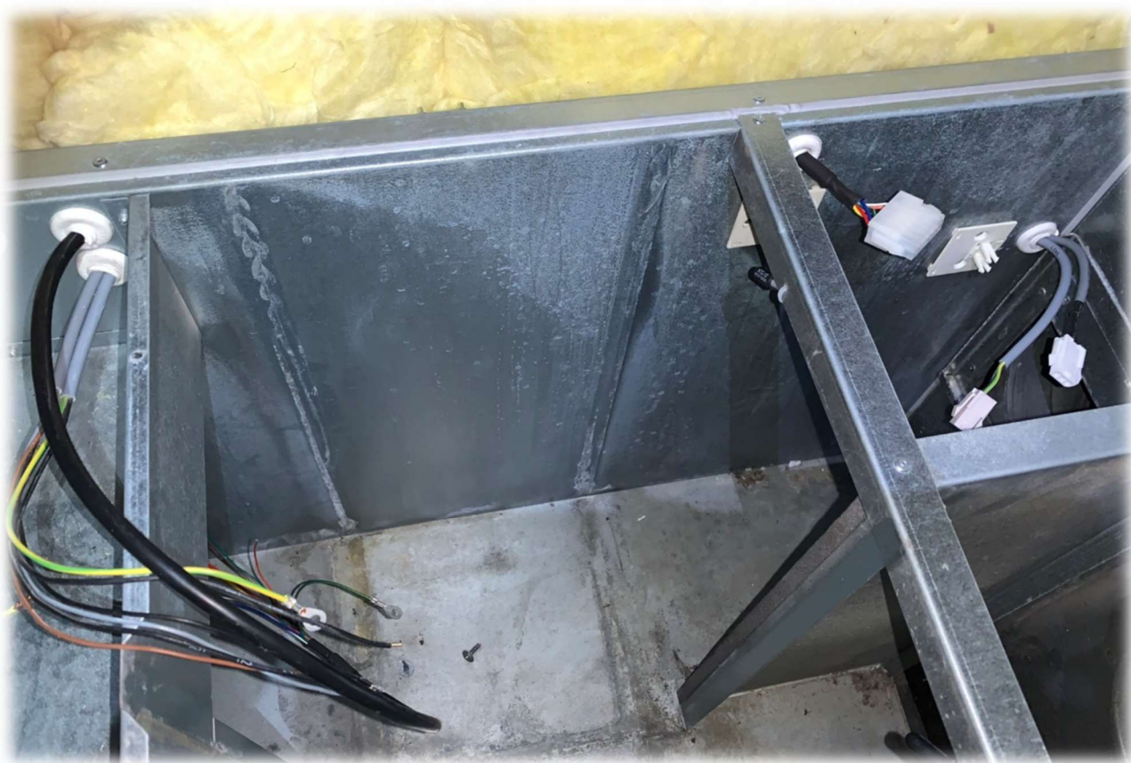
New cables installed.
