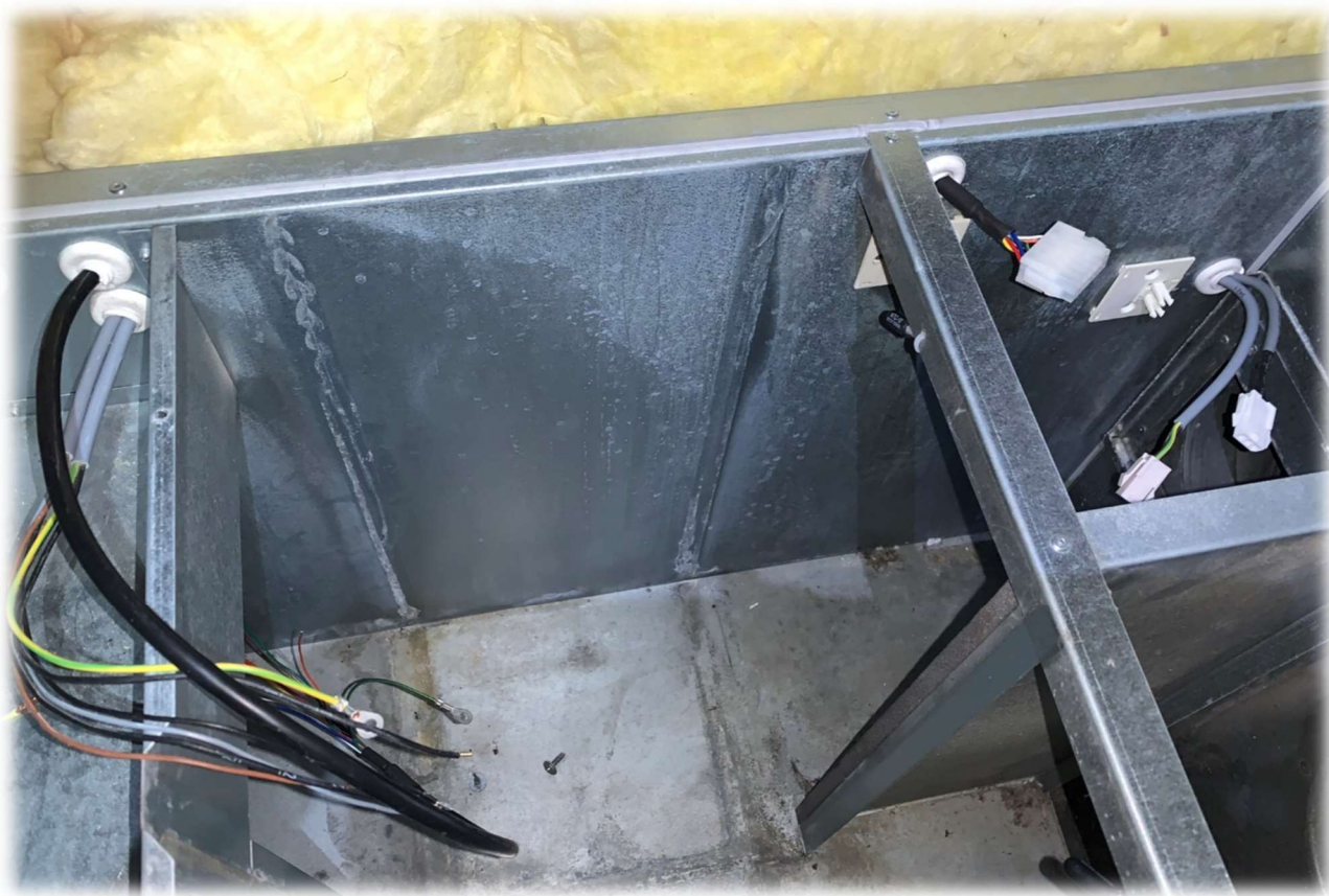
New cables installed.
