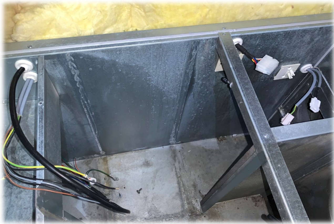
New cables installed.
